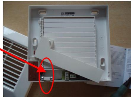
2. Connect the fan with power supply using the terminal strip. Usually goes from wall electric cable with 3 wires, so the blue is directly earthed conductor (N), brown / black is the phase conductor (L – under constant voltage) and third yellow-green is the circuit protective conductor (no need to connect when mounting plastic fan, can be blinded). Install the fan so the service cables will be in lower part of the fan.
